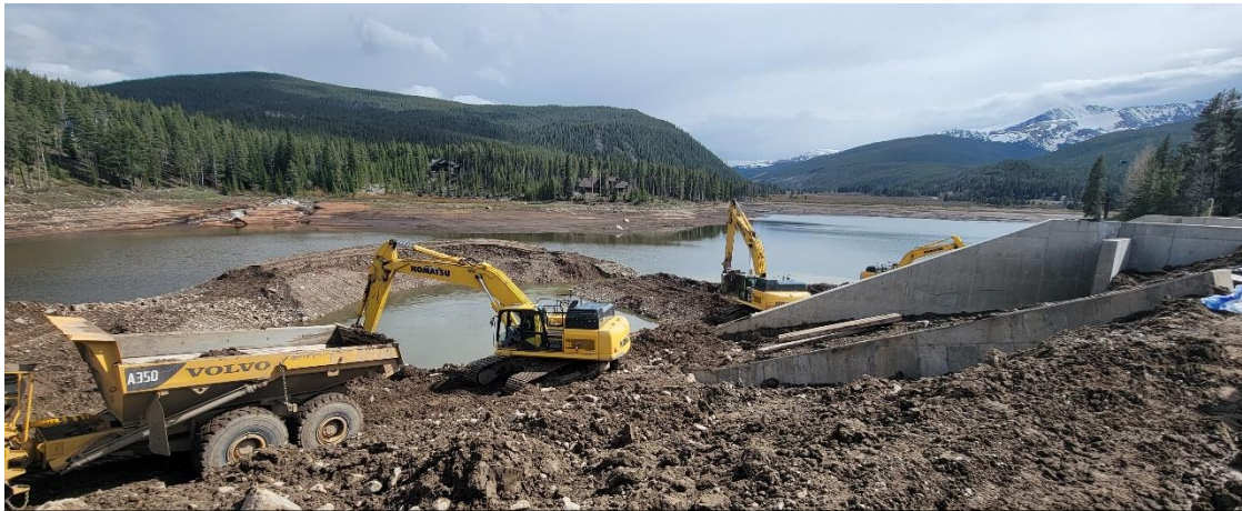
Crews begin removal of the cofferdam.
