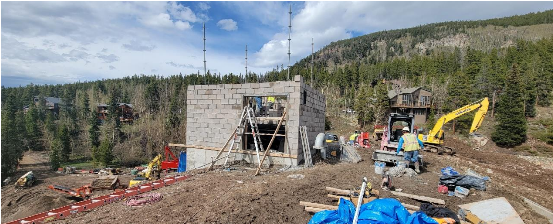
The new control house under construction.
