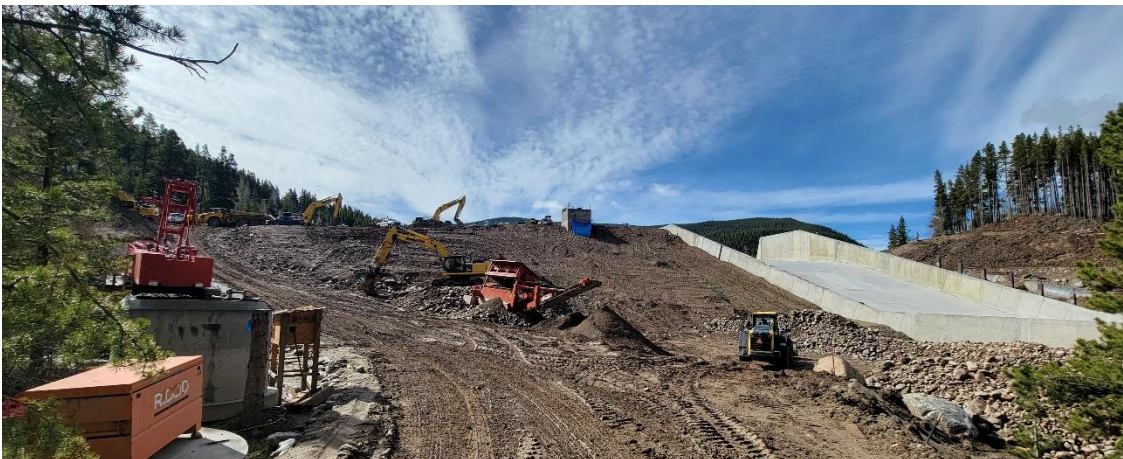
Grading on the east side of the dam.
