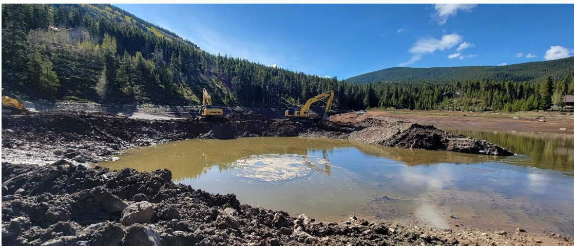
Progression of cofferdam removal.
