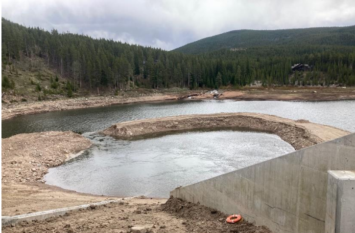
Controlled breach of the cofferdam to equalize water levels prior to beginning excavation.
